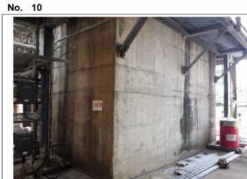
Tag/ part M1-423, Dryer support Finding Normal Condition
