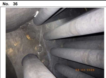
Tag/ part M1-423.baffle plate Zone I Finding Moderate corrosion was found on baffle plate .
