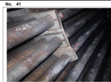
Tag/ part M1-423.baffle plate Zone D Finding Damage Baffle already repaired
