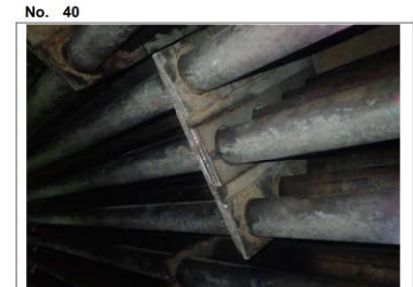
Tag/ part M1-423.baffle plate 13 Zone D Finding Damage Baffle already repaired
