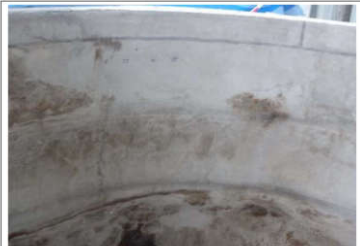
Tag/ part M1-423.Stack Finding Slight corrosion was found on shell
