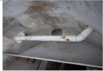
Tag/ part M1-423.Stack Finding Slight corrosion was found on shell and coating damage on the inlet nozzle.
