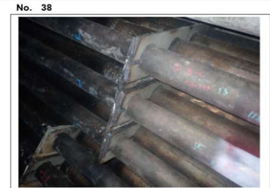
Tag/ part M1-423.baffle plate Zone B-C Finding Damage Baffle already repaired
