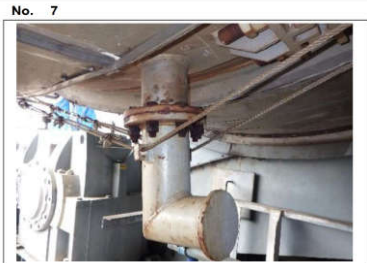
Tag/ part M1-423, Nozzle Finding A minor rust stain was found on the nozzle.
